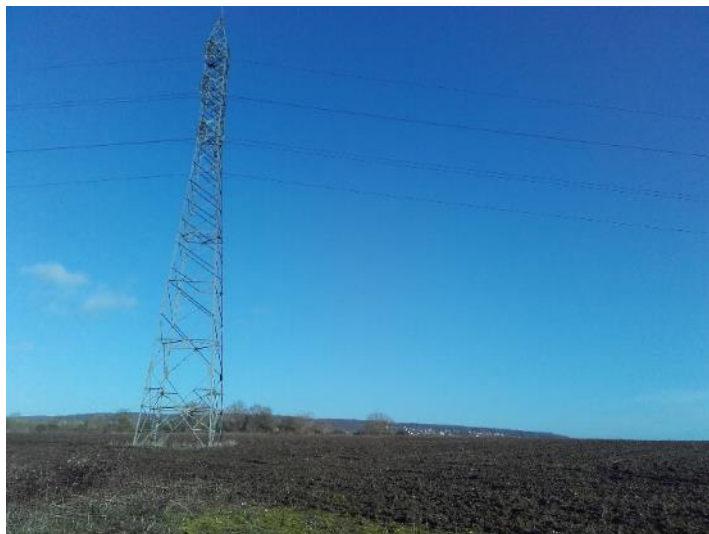
Figure 13 – Photo 7 - Ligne Haute-tension (Source : GPS&O)
